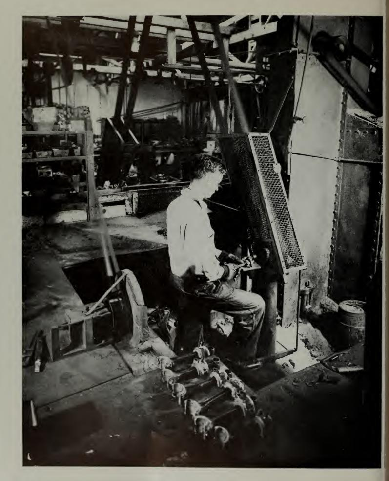
Then the steel separator shims are removed by the means of the socket wrench shown in picture number five, and any auxiliary nuts and bolts are removed and the originals replaced.
